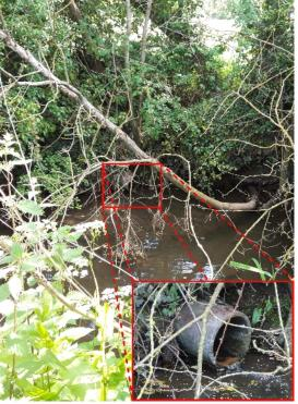
Photograph 10 - Highway drain outfall into Poulton Brook
